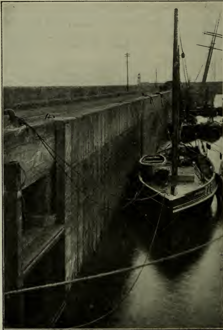
REINFORCED CONCRETE AT NEWLYN HARBOUR.
